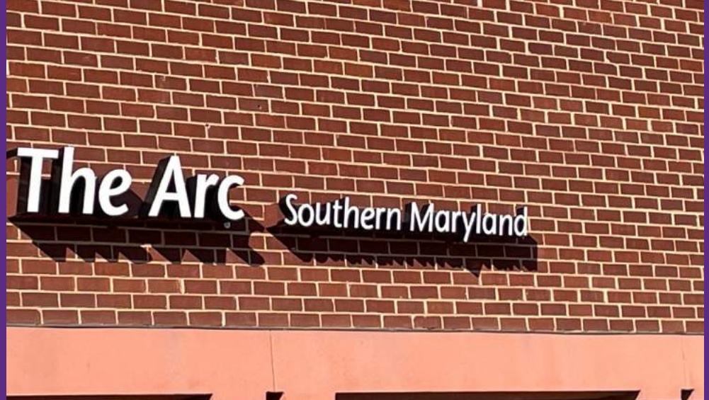
PICTURED: LOGO SIGN BEING INSTALLED AT NEW OFFICE
